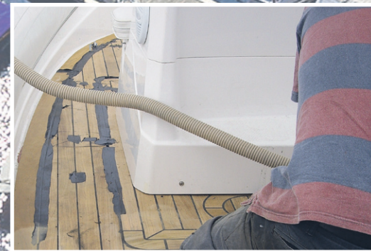
Installation service $110sqm
