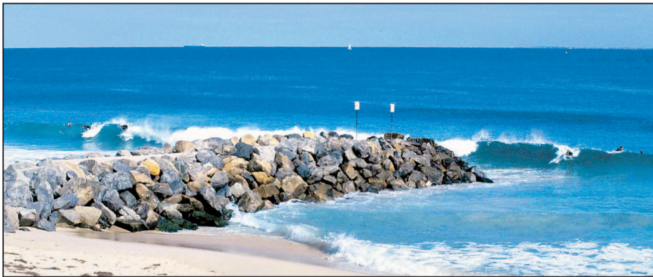
An extension to Floreat groyne has been suggested as a way to alleviate erosion and create waves for local surfers. Picture: Luke Simon.
