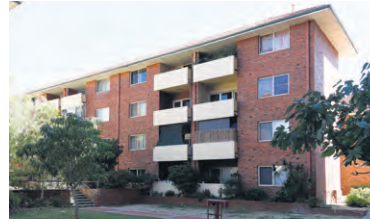
Enclosed balconies at Wandana are to be removed.
